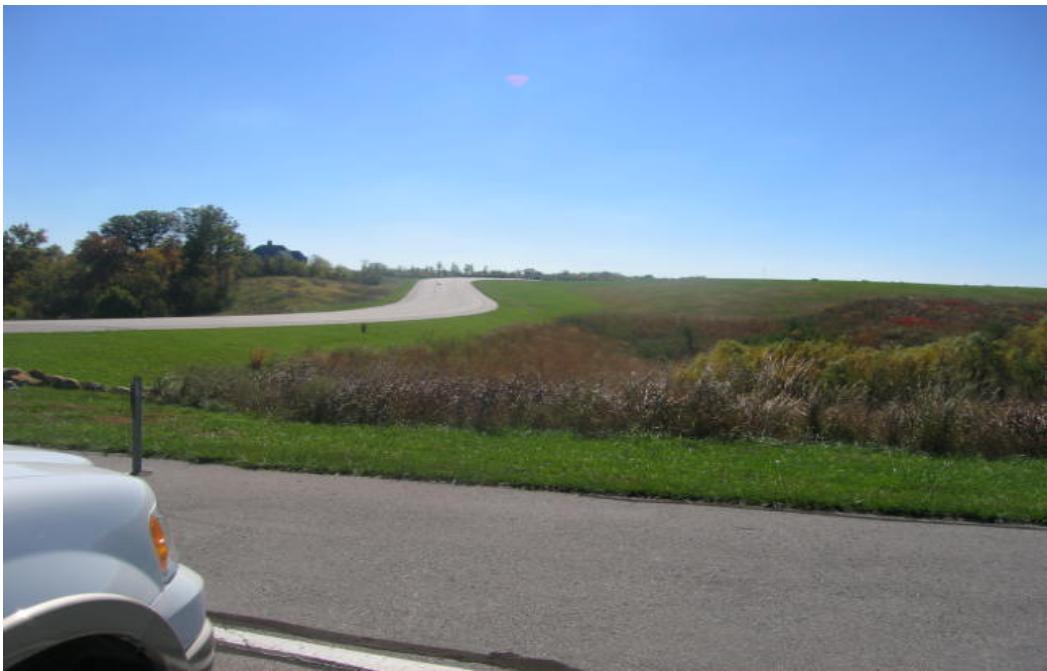
View South along Valley Parkway
